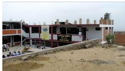
New wing of CETPRO of Alto Trujillo dedicated in June
